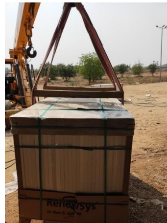
Fig: Packing Box –Adjusting Sling rope for Hoist Handling (Separator – Wooden Plank)
