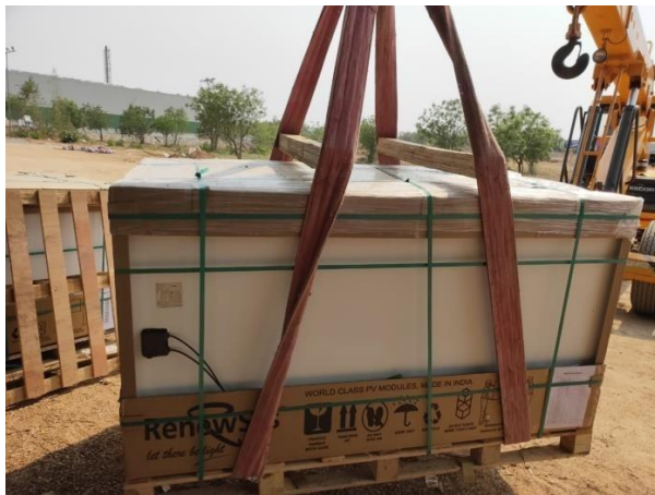
Fig: Packing Box –Adjusting Sling rope for Hoist Handling (Separator – Wooden Plank)
