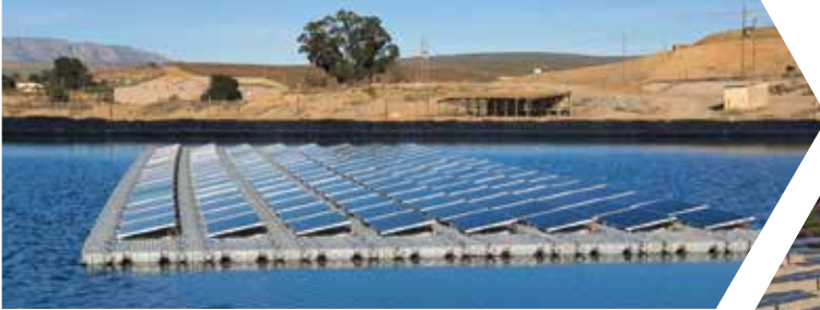
Floating Solar Plant, Cape Town, SA
