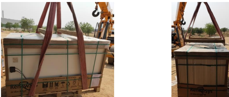
Fig: Packing Box - Adjusting Sling rope for Hoist Handling (Separator – Wooden Plank)
